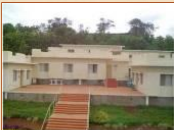
(above) Old dormitories 1,2,3
