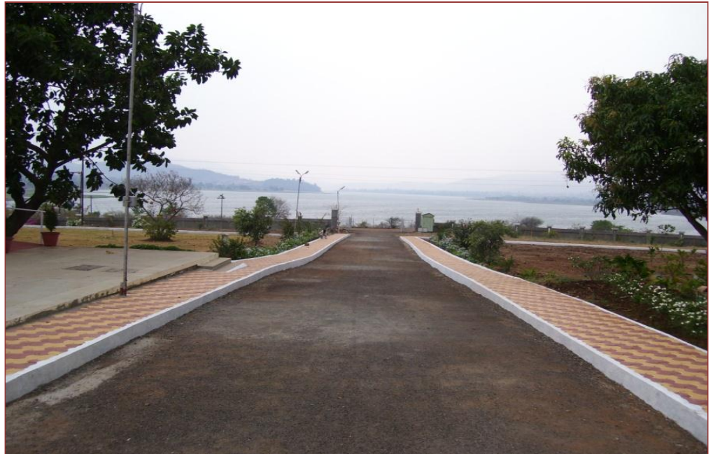
(above) Newly constructed pathway at Pune Retreat Centre
